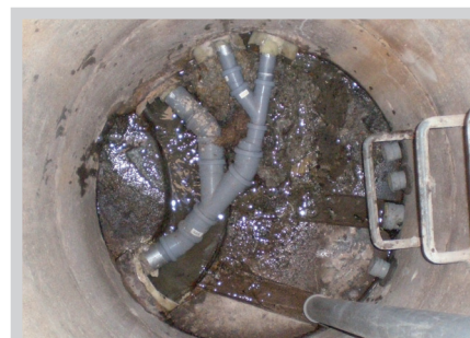
connections in manhole
