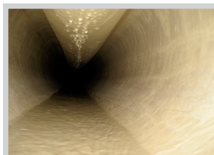
interior view of a rehabilitated XTRA liner segment
