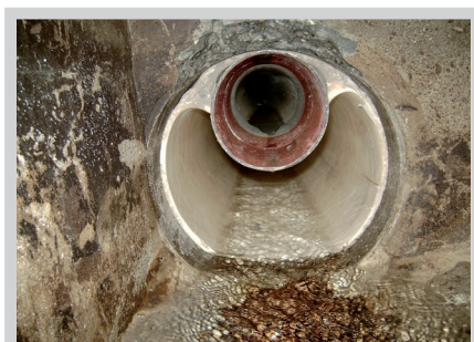
XTRA liner after rehabilitation
